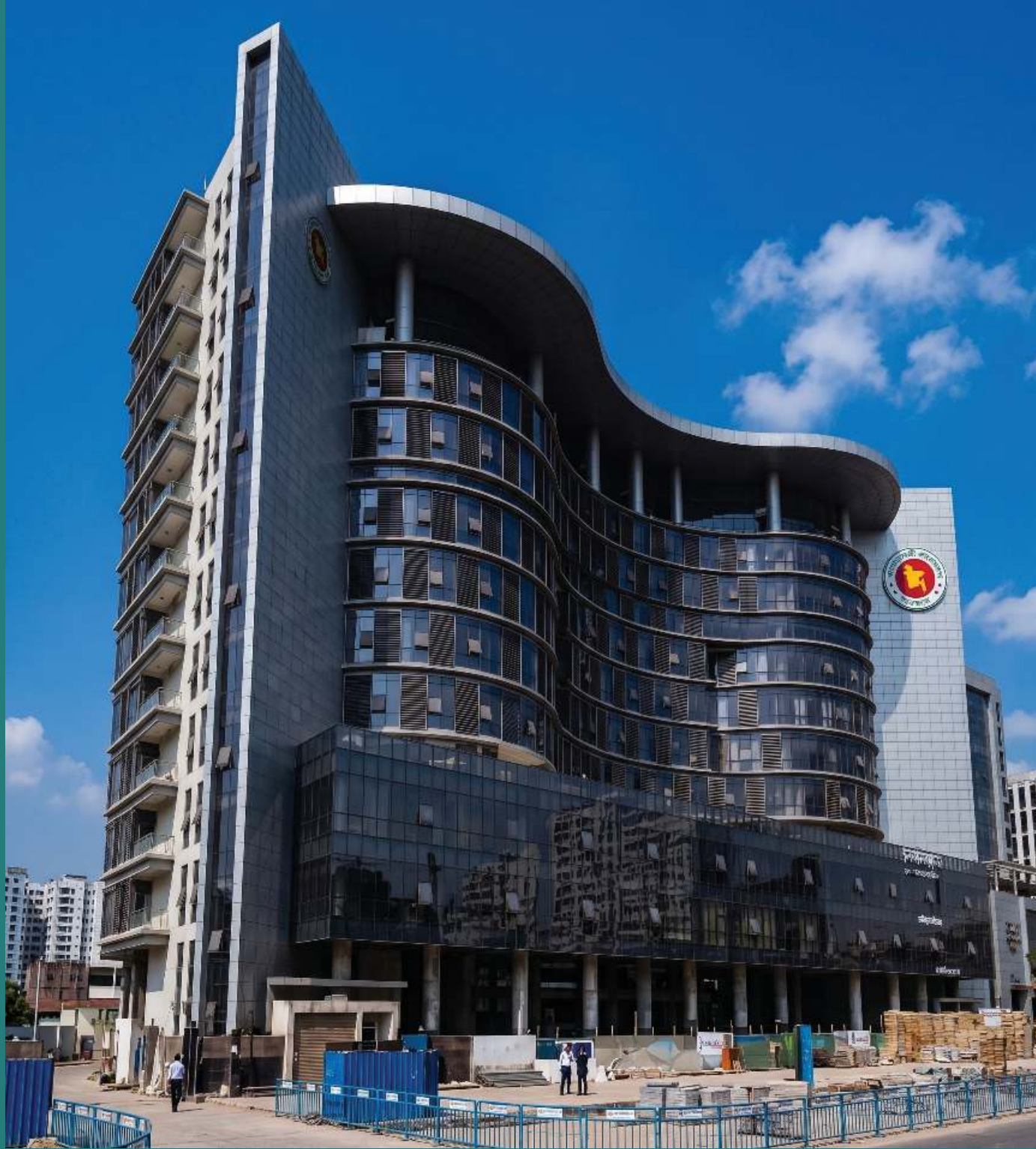
Name of the Project with Location: Construction of Bangladesh Telecommunication Regulatory Commission Building 12-storied with 3 Basement considering 15 story Foundation) at Sher-e-Bangla Nagar, Dhaka. Including Civil, Sanitary, Internal Electrification etc. under Public Work Department
